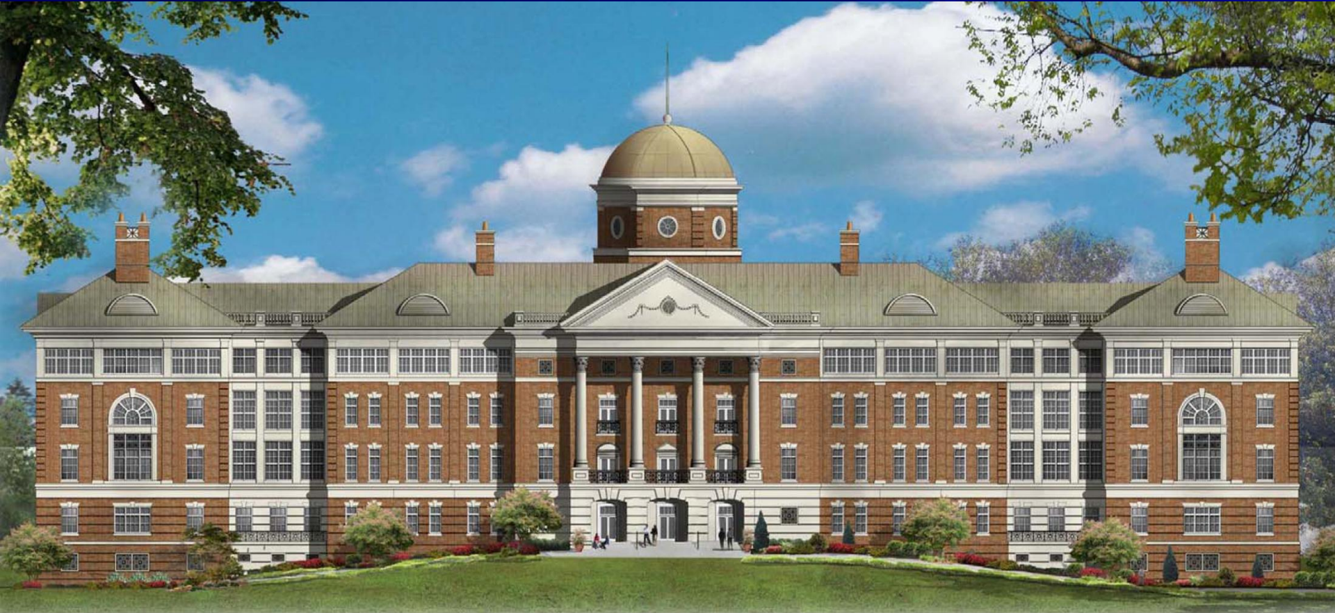
CORE LABORATORY BUILDING
